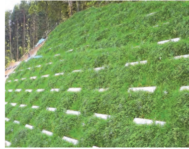
LL 補強土工の工事例
